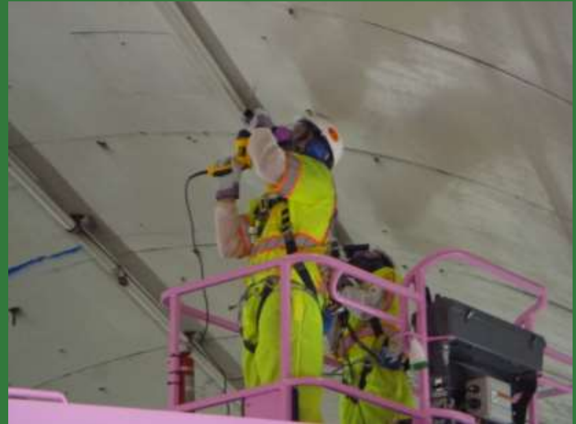
Drilling into ceiling
